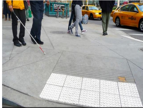
Tactile warning on a curb cut on a sidewalk. Individual with a white cane in the background.
