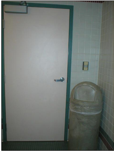
Toilet room – room where people enter and exit unsupervised
