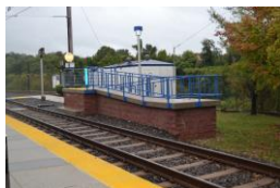
Maryland MTA Light Rail "Mini-High" Platform to allow boarding by wheelchairs users and other unable to climb steps onto high floor light rail cars.
